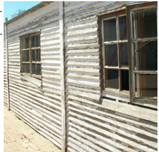
Peeling paintwork on classroom buildings - now fixed!
